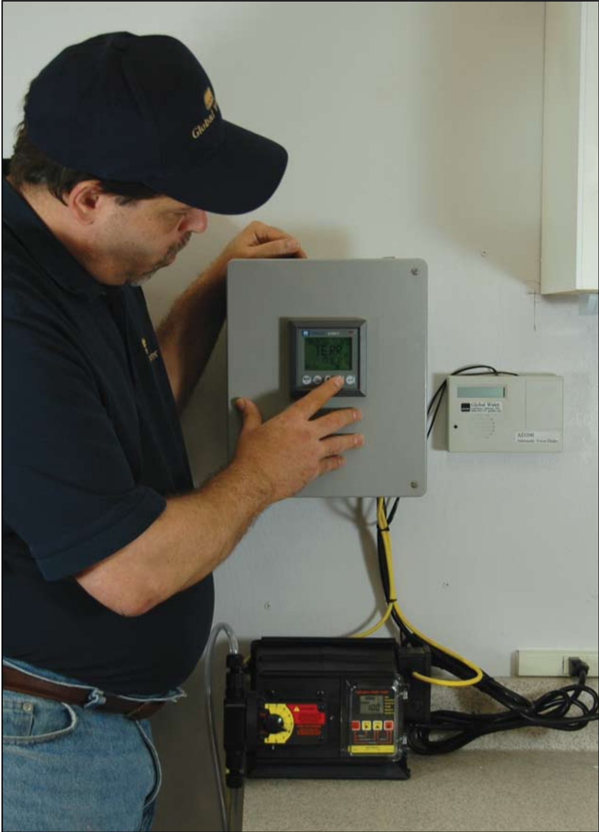
Easy voice alarming with Global Water's AD200 Voice Autodialer, shown here with a pH/ORP Controller and a chemical metering pump.
